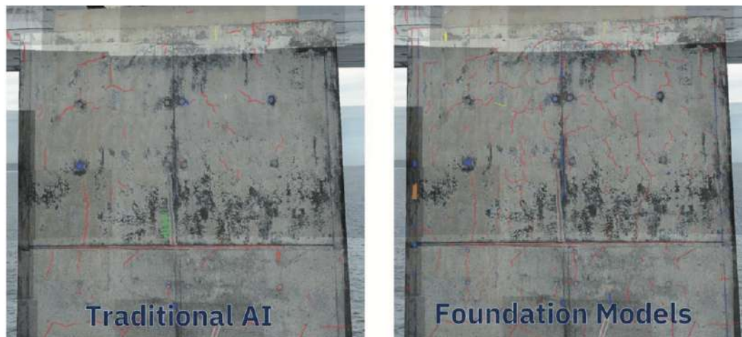
Figure 1: Comparison of AI outcomes on the south face of Storebaelt Pillar 3. On the left: results from traditional supervised learning. On the right: results from a foundation model (FM)
